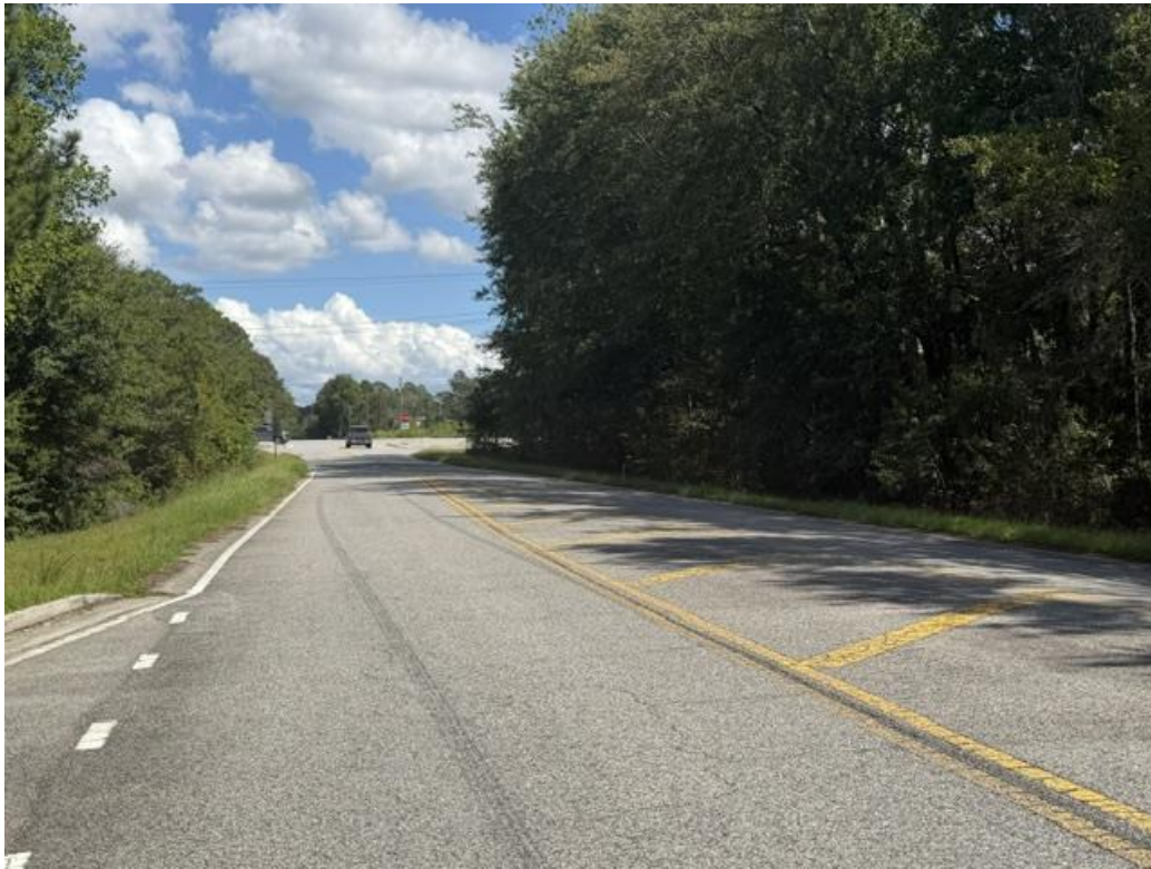
View of the properties from the ROW on West Jones Mill Road, facing east.
